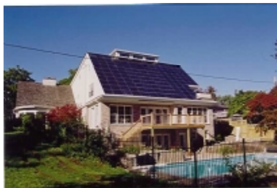
Figure 2. ARISE HOME Research and demonstration covering the surface of this rooftop with both solar thermal and 5kW of PV panels. The objective is to develop a comprehensive solar energy system that will provide much of the electricity and heating needs for new homes. (Photo: ARISE Technologies Corp.)
