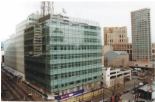
Figure 3. The renovation of this 52-year-old building incorporated a new façade that provides waste heat recovery and the 2.5kW PV panels now power DC fans that ventilate this air space. (Photo: BCIT)
